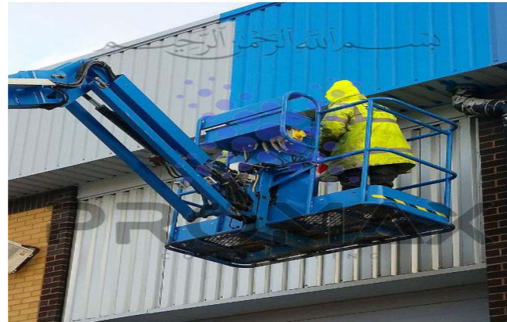
INDUSTRIAL GRADE EXTERNAL / INTERNAL PAINT WORKS Pg. 33 to 36
